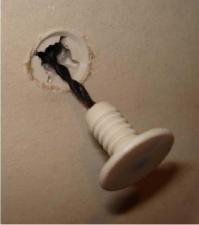
7. Use your thumb to carefully push the sensor body into the threaded outer case until the face of the sensor body is flat against the drywall. See figure below.
