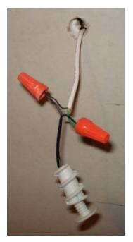
5. Carefully feed the wires and wire nuts through the ½ inch hole and into the wall. Use your fingers to start screwing the threaded outer case into the hole in the wall as shown on the right.
