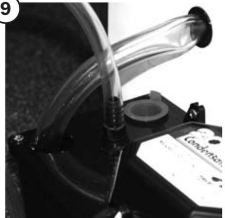
Route the condensate pump drain hose to an appropriate drain and plug the condensate pump into a standard 115VAC outlet.
