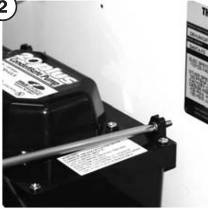
Pre-drilled mounting holes are located near the bottom and on the same side of the unit as the drain hose.
