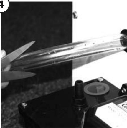
Cut the condensate drain hose at a 45° angle approximately 10 inches from the unit.
