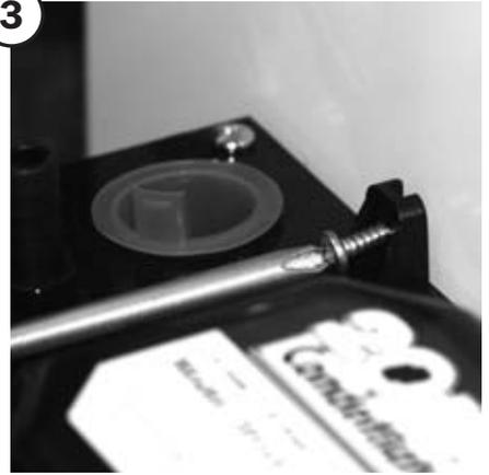
Secure the condensate pump to the unit with the two provided screws.
