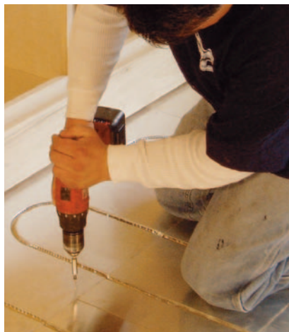
SCREWING INFLOORBOARD™ BOARDS
