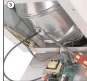
Remove the relative humidity sensor cover.
