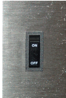
Figure 10: Vehere fan switch.
