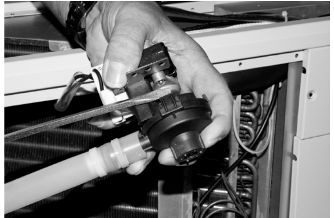
Fig. 7: Use a screwdriver to pry open the impeller housing retaining tabs.
