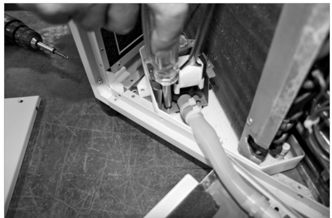
Fig. 5: Remove the four pump bracket bolts from the CMC drain pan.
