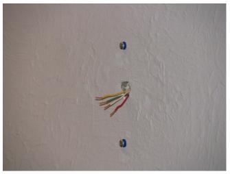
Wall mounting location with the existing thermostat cable prepared to install the new Thermostat Keypad.
