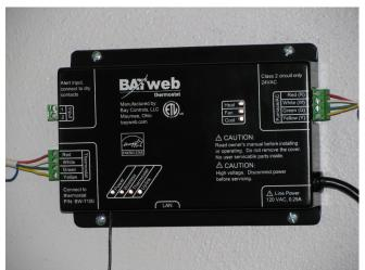
The Control Module installed and wired to your furnace/air conditioner.
