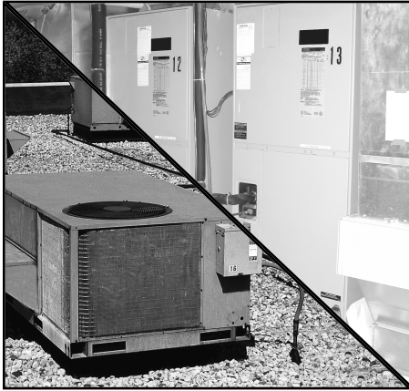
HVAC Equipment Split System
