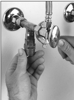
2. Install tees and attach angle stops.
