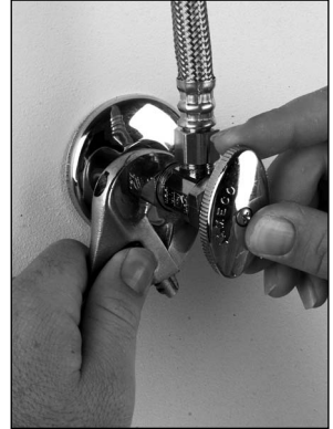
1. Turn off water supply and remove angle stops.
